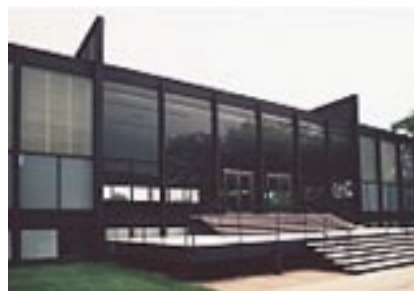
Figure 1 Crown Hall, at the Illinois Institute of Technology (IIT)
