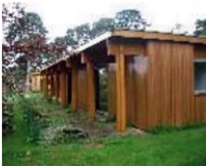
Figure 2 'Teesdale' – Grade II listed existing house in Surrey
